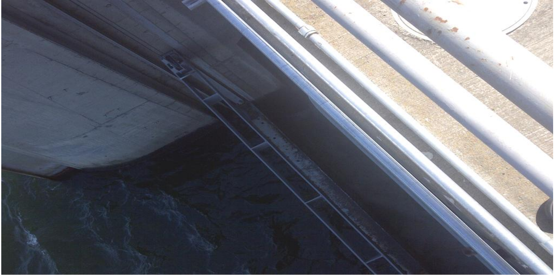
New lift beam with recessed bars installed at sluiceways 1-2 and 1-3.
